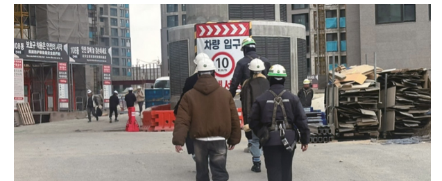
Construction Site Tour
